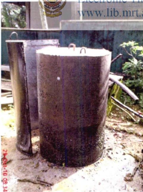
Presently used meshed concrete block pre cast at site to obtain a smooth surface
