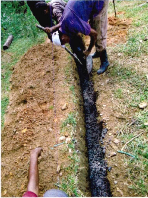
Covering the horizontal cable part with conductive concrete mixture
