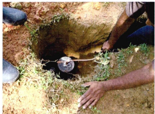
Laying the horizontal cable part
