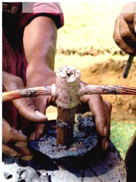
Exothermic Welding of the copper Conductor
