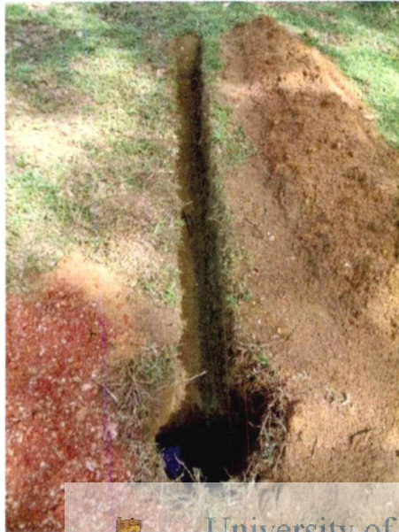
Pit dug for installing the earth
