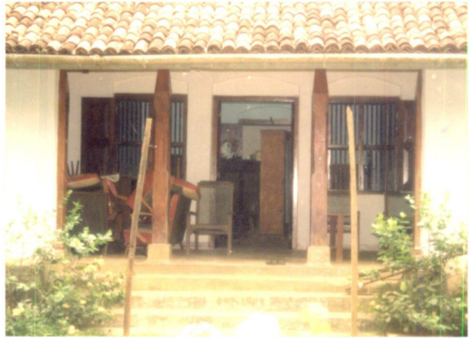
Fig.2.15. Openings were placed so as to cut down the solar radiation coming in to the building
