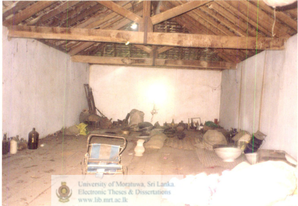
Fig.2.3. Roof is a very dominating element in traditional house
