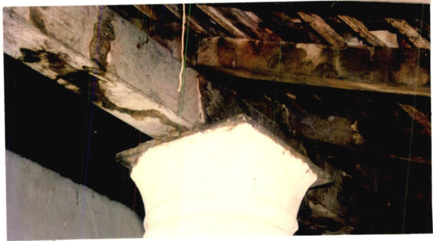
Fig.2.18 The gap between roof and the wall provides the good air circulation.
